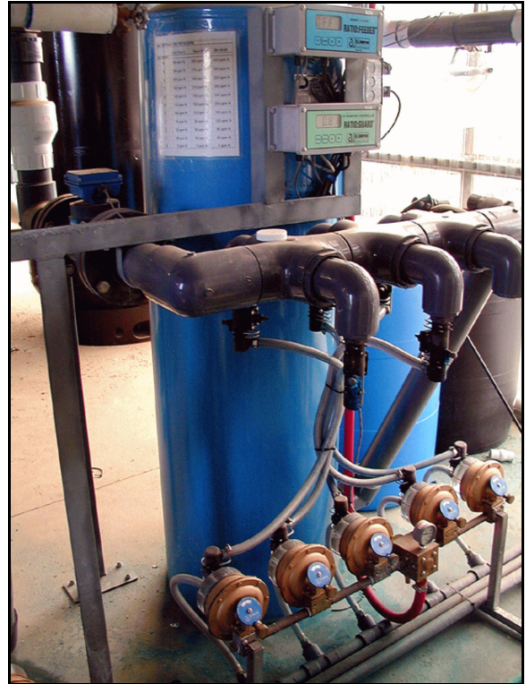
Figure 5. H.E. Anderson injector with multiple fertilizer injector heads.
